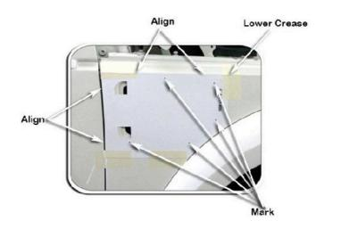
Drill a pilot hole for each marked hole positions.
